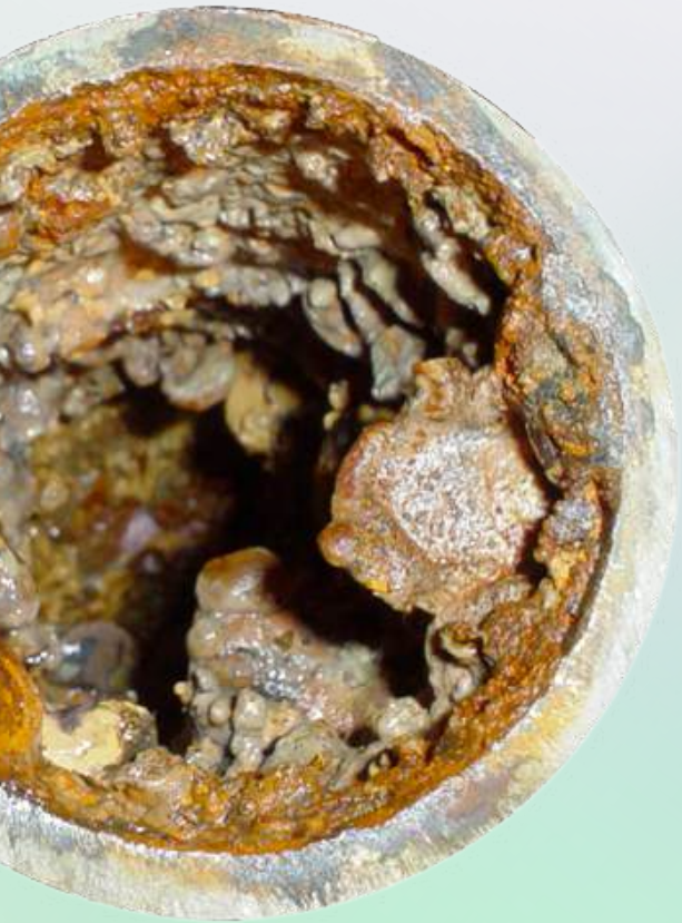
Water Lead Pipe
